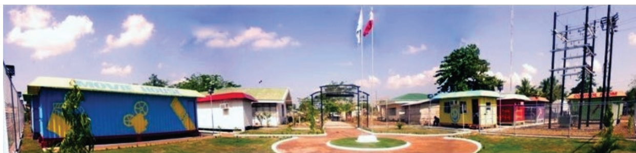
Panoramic view of Powersource Philippines' Power Plant Facility (Photo Credit: PowerSource Philippines Inc.)
